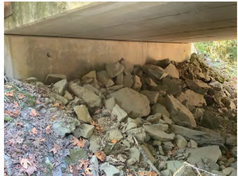
Left Bank Abutment when facing downstream
