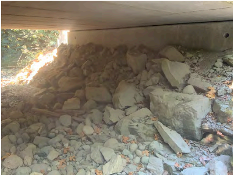
Right Bank Abutment when facing downstream
